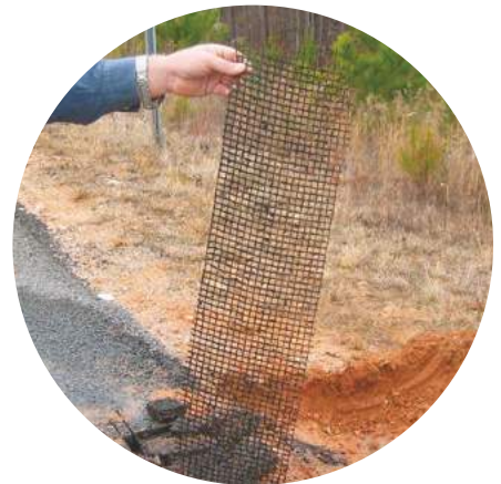
ADFORS GlasGrid carefully removed from the pavement after 5½ years with no damage
