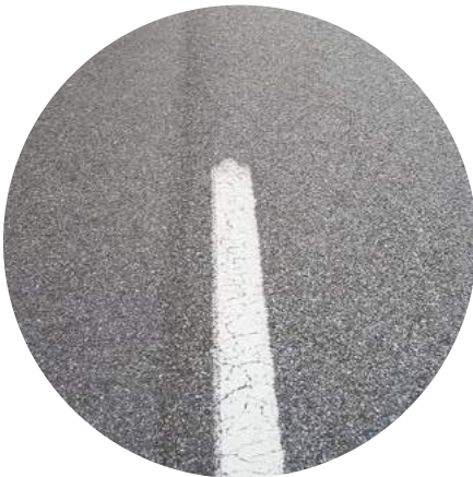
Section with ADFORS GlasGrid shows no cracking
