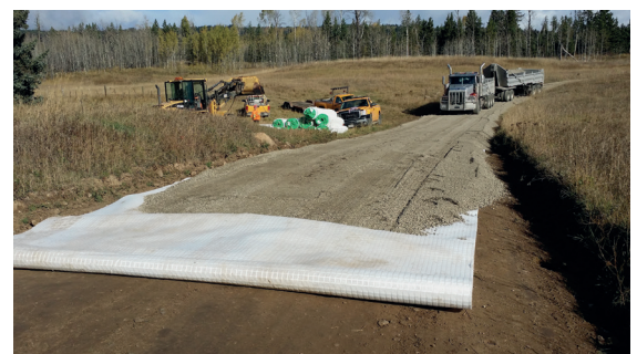
Figure 7: Combigrd® and Secugrid® installation
