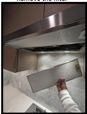
Remove the filter
