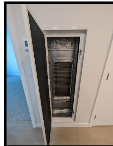
Remove and Replace Filter
