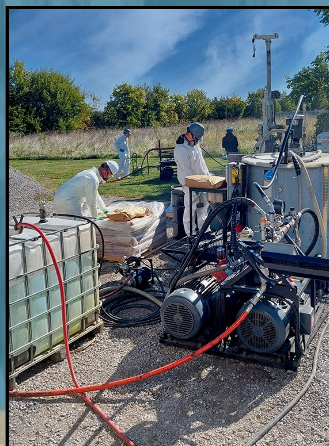
Figure 2. Example of Injected PRB
